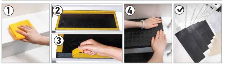
Before installation, the stairs must be cleaned. Sweep the stairs with a broom to remove dust & dirt, wipe clean and dry with a lint-free cloth.
